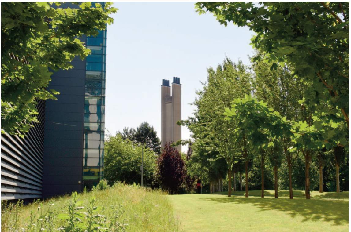
Image 5: Addenbrooke's Hospital incinerator chimney Image Credit: CBC Ltd
